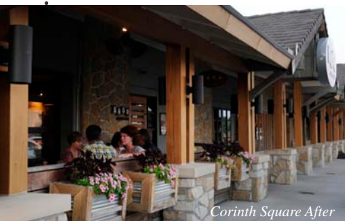
Corinth Square After
