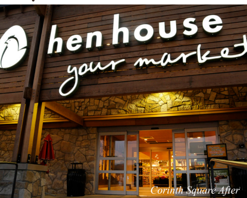
Corinth Square After
