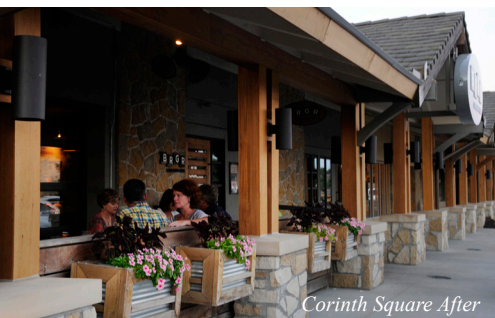
Corinth Square After
